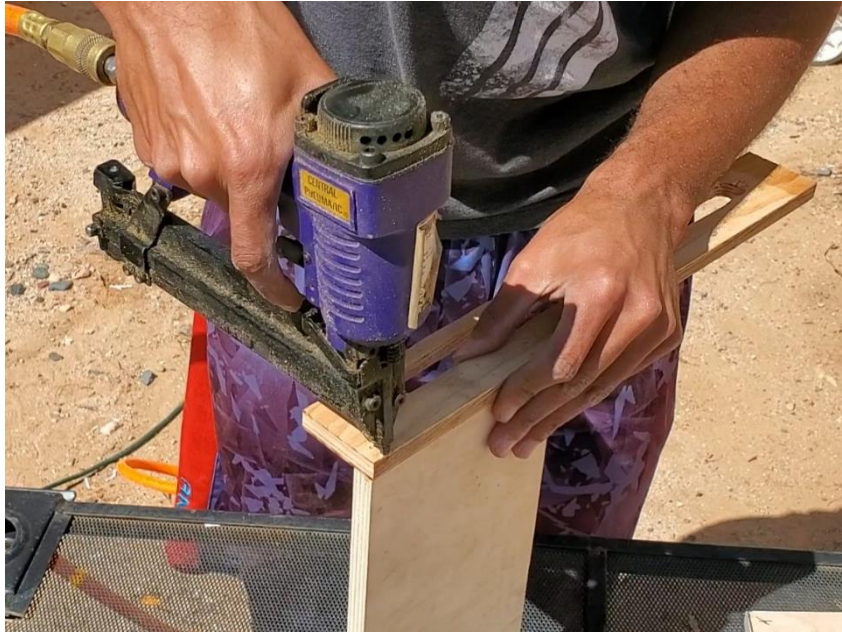
Figure 8: Stapling the side rails
