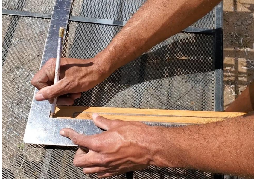
Figure 4: Marking out the slot location
